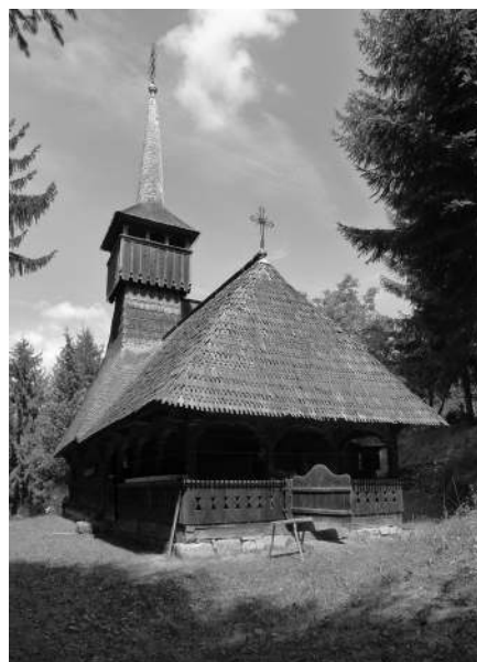
Wooden church of Călinești Căeni, view towards supersized porch.
